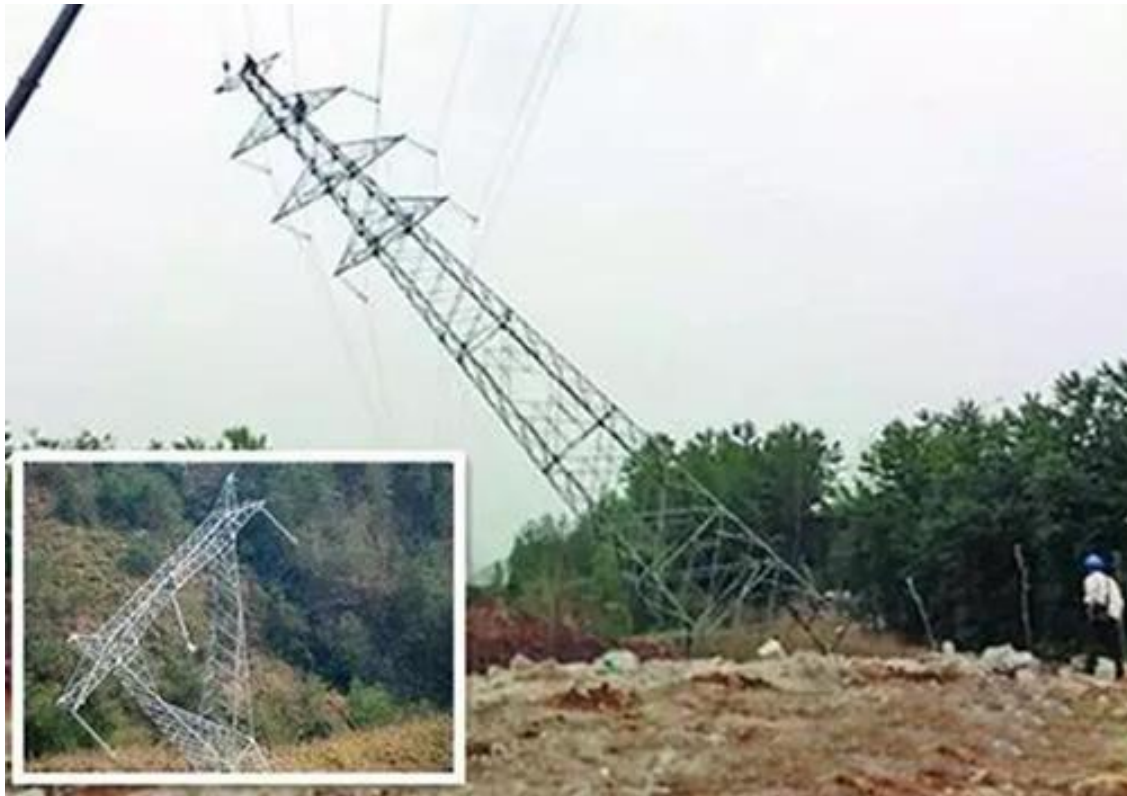
Figure 2: Typical Transmission Line failure in many places
