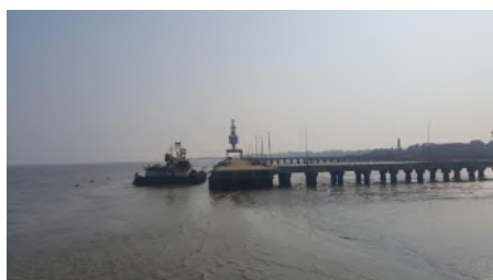
Fig.10 View of Kaladan Multimodal Transport Project at Sittwe
