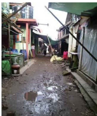
Fig.16 Narrow Spacing between Buildings' Facade to Facade
