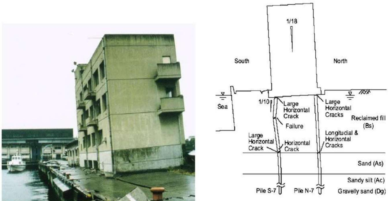
Figure 2: (a) Tilting of a pile-supported building following the 1995 Kobe earthquake; (b) formation of crack. (Source: Bhattacharya, et al. [8]).
