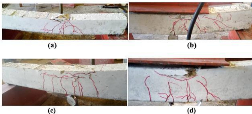
Figure 4. Crack Pattern of study samples: (a) Type-BC, (b) Type-B1, (C) Type-B3, and (D) Type-B2
