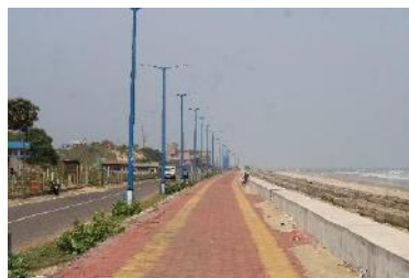
Fig 22: Violation of CRZ norm
