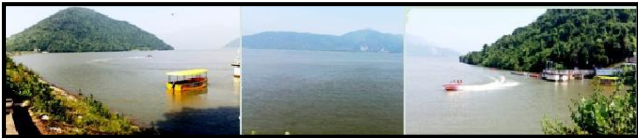
Fig 1. Overall view of Tatipudi Reservoir
