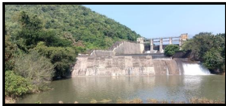
Fig 3. Outlet view of Tatipudi Reservoir
